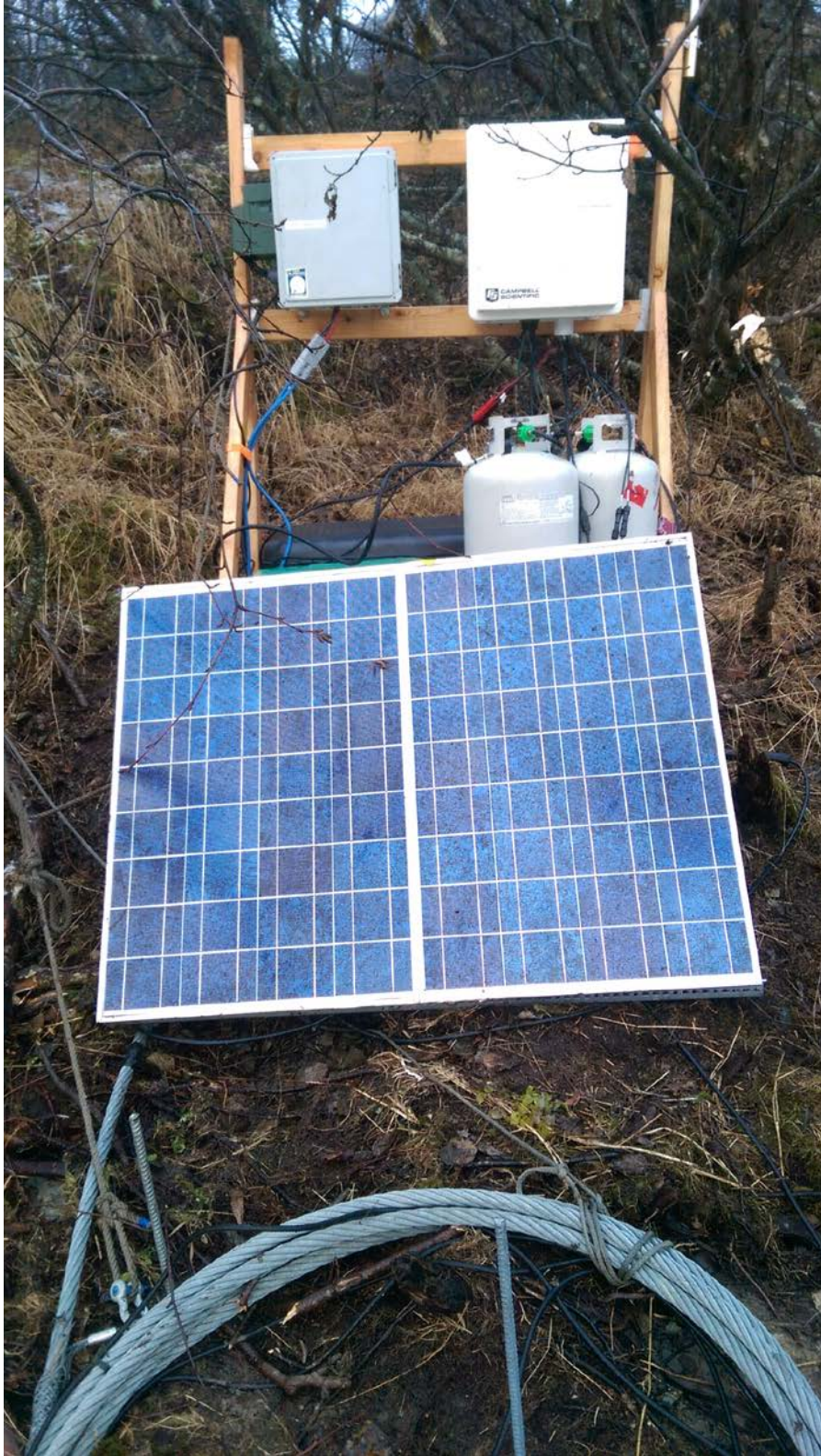
Figure 33. Power System with Solar Panels, November, 2016.
