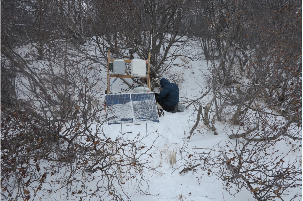
Figure 38. UAF personnel working on the remote power/real-time data telemetry system in February, 2017.
