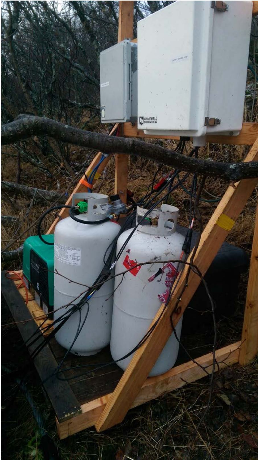
Figure 34. Remote power and data telemetry system, November, 2016.
